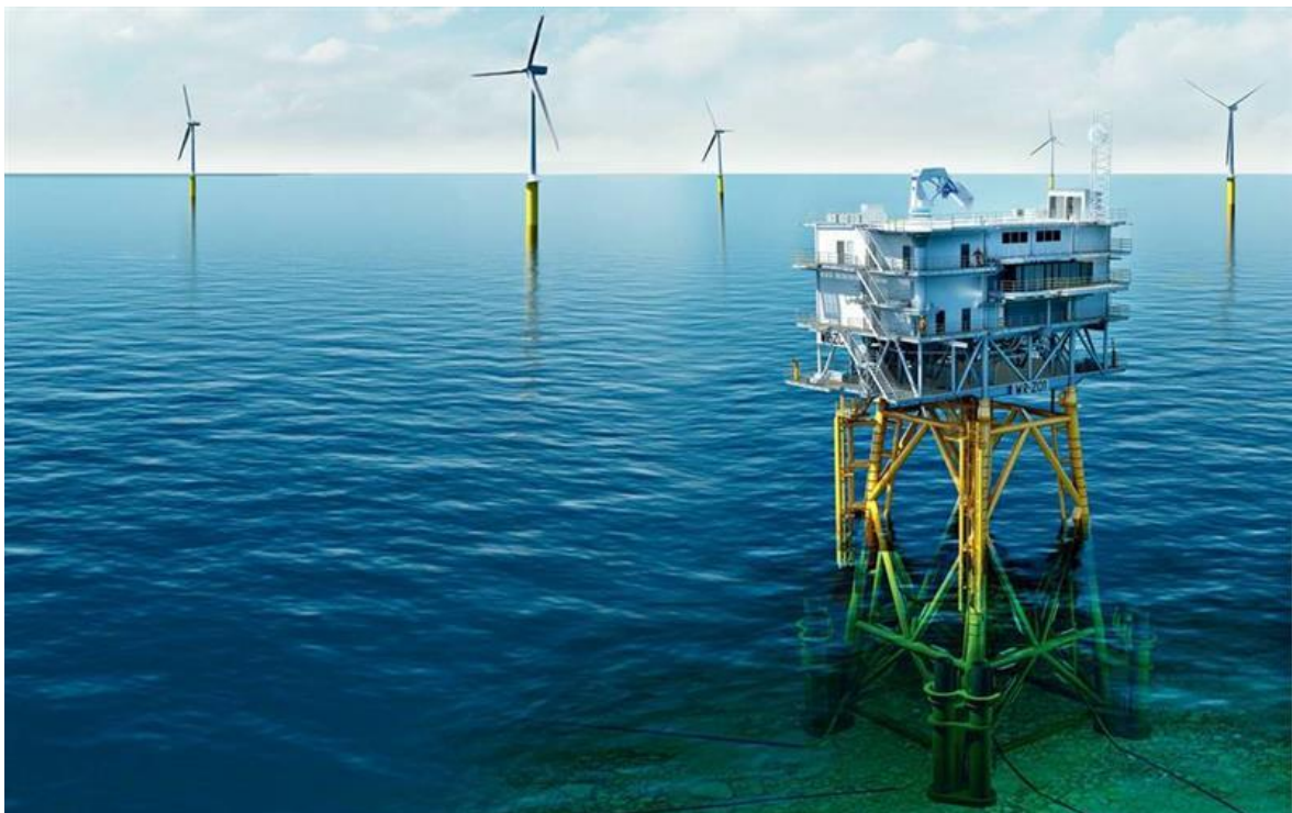
Abb. F.3: Offshore Sub Station © Ramboll 2021
