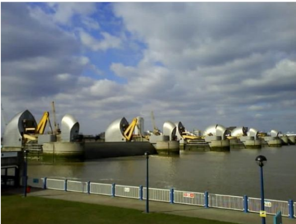
Figure A 5: Thames Barrier
