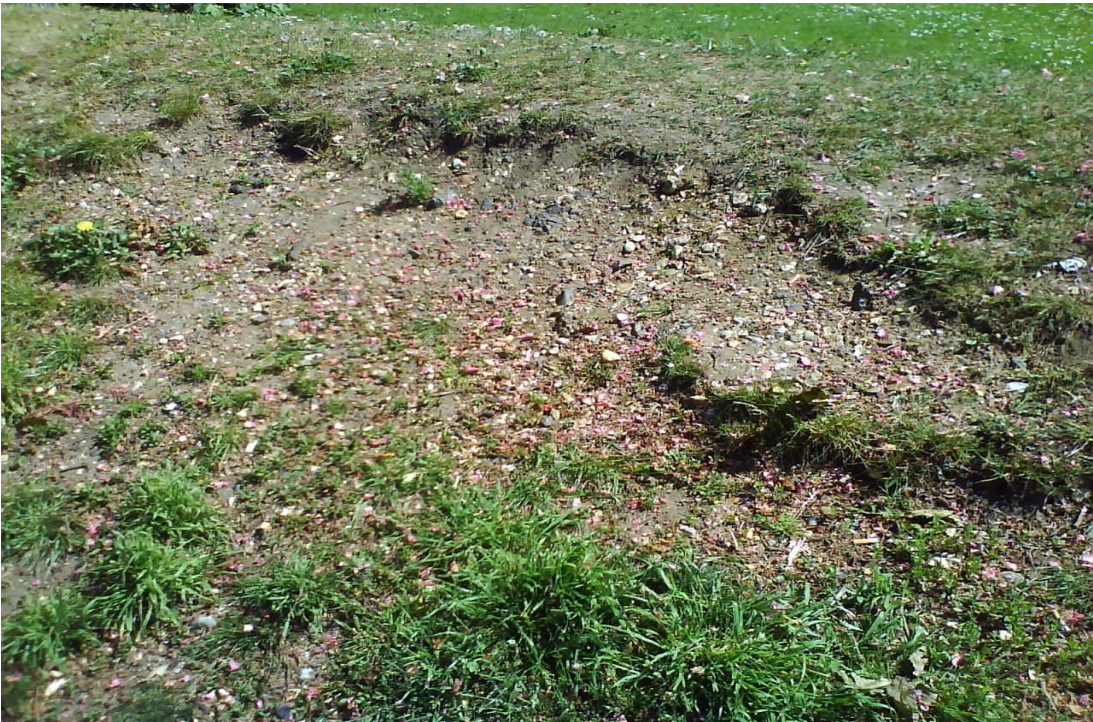
Figure A 20: Green bunded defence destroyed through walking over the defence.
